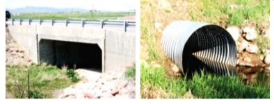
Figure 11: Concrete box culvert and corrugated metal pipe.
