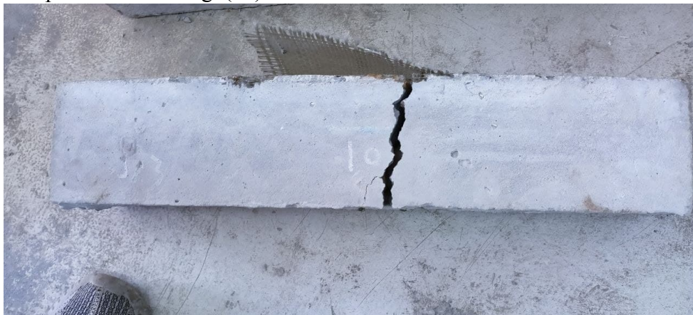
Fig. (15): Failure shape of S15
