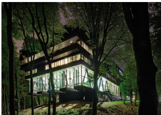
Figure 3: The building's direct connection with nature in the forest
