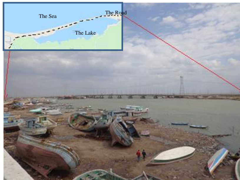
Fig. (5): The penetration of the international road and the high-pressure towers in the lake inlet.
